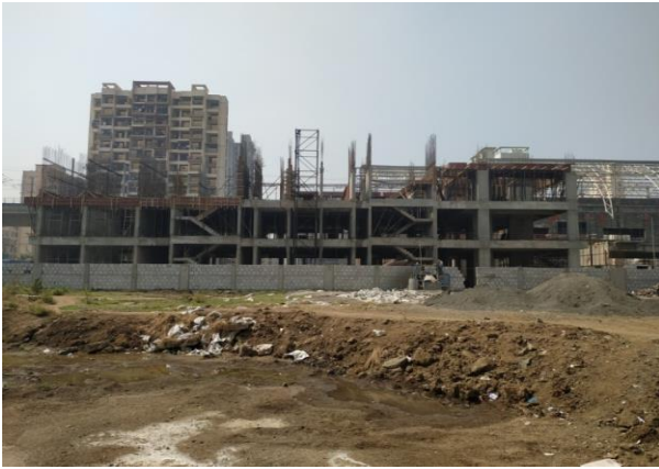
Figure 2: Construction Site at Mumbai
